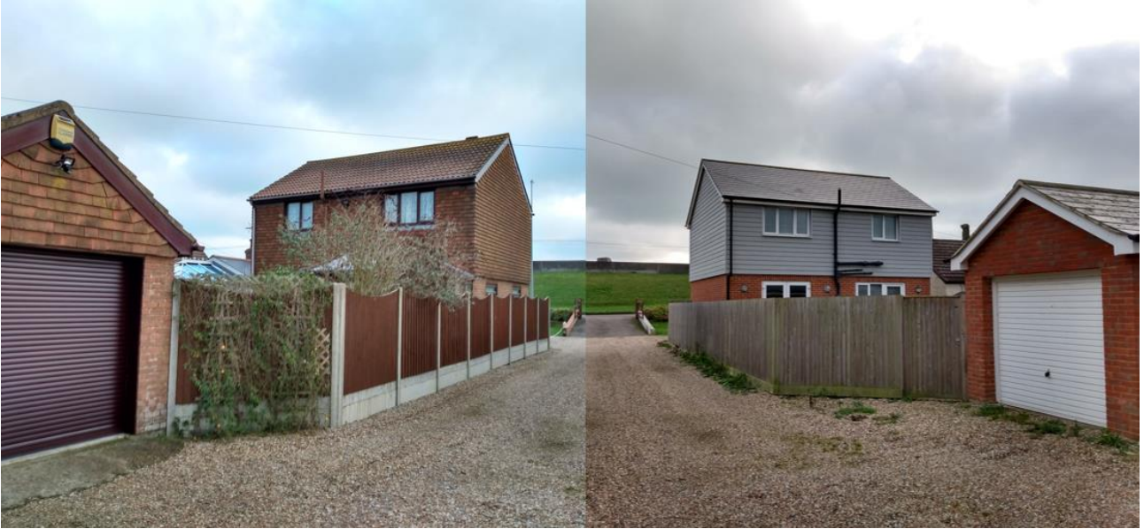
Photo 4: Rear of 1 and 2 Willop Close
